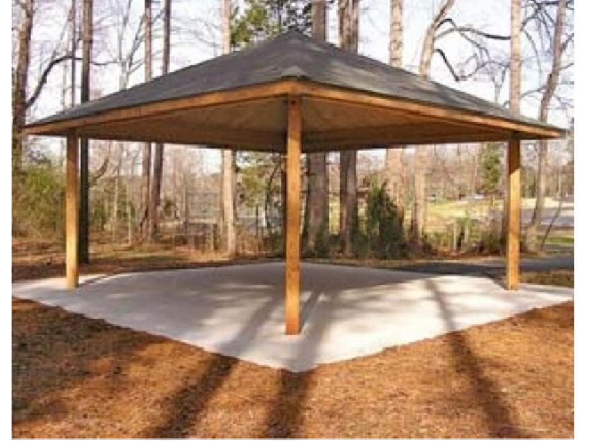
IMAGE ABOVE: TYPICAL WOOD OUTDOOR AMENITIES STRUCTURE WITH CONCRETE PAD. THIS PAVILION SERVES THE SIMPLE PURPOSE OF PROVIDING SHADE AND COVER FROM THE ELEMENTS FOR RECREATIONAL USERS. PICNIC TABLES SHALL BE LOCATED HERE TO PROVIDE SEATING, AND SHALL BE CONSTRUCTED OF THE SAME BUILDING MATERIAL AS THE PAVILION. ADDITIONAL AMENITIES TO BE LOCATED IN THIS AREA: COMMUNITY INFORMATION BOARD, BENCHES, AND REFUSE CONTAINERS.
